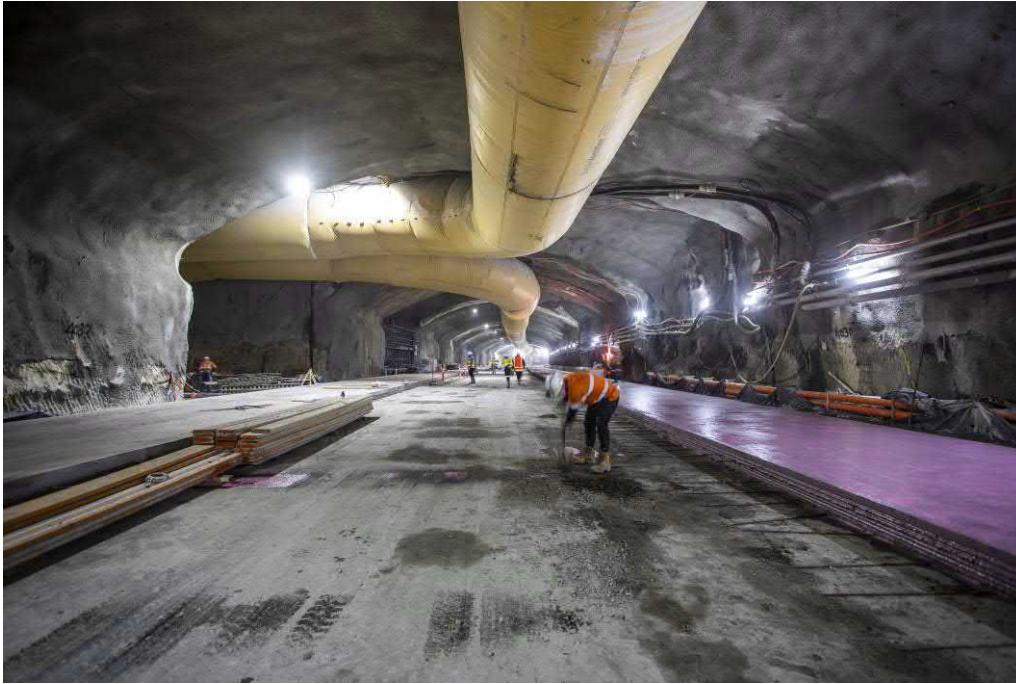
Figure 2-1 - Continuously Reinforced Concrete Pavement (CRCP) paving works at PBR in July 2020
