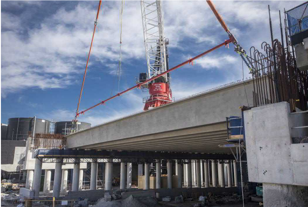
Figure 2-3 - Super T installation at Campbell Road
