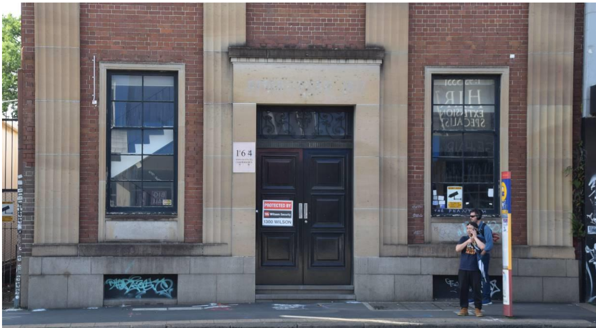
Photograph 3: Lower portion of main elevation
