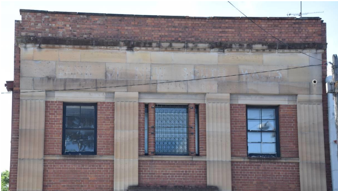
Photograph 2: Upper portion of main elevation
