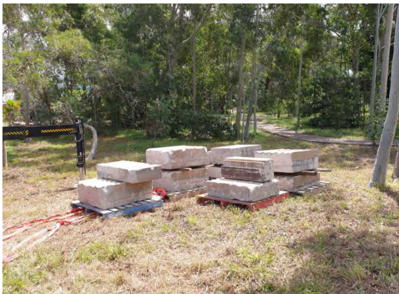
Figure 4-2 Salvaged items at Wilkins Public School for beneficial reuse
