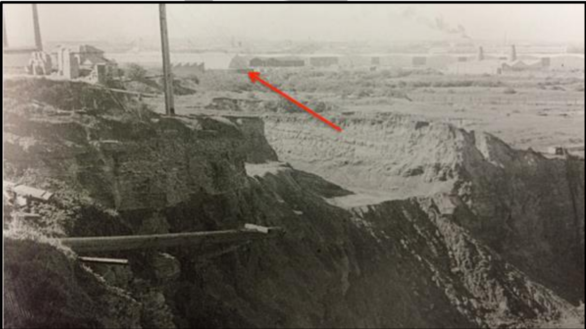
Figure 4 – The Austral pit which was shared by The Central Brick & Tile Co Pty Ltd. The first building on the subject site can be seen in the background (indicated by red arrow).
