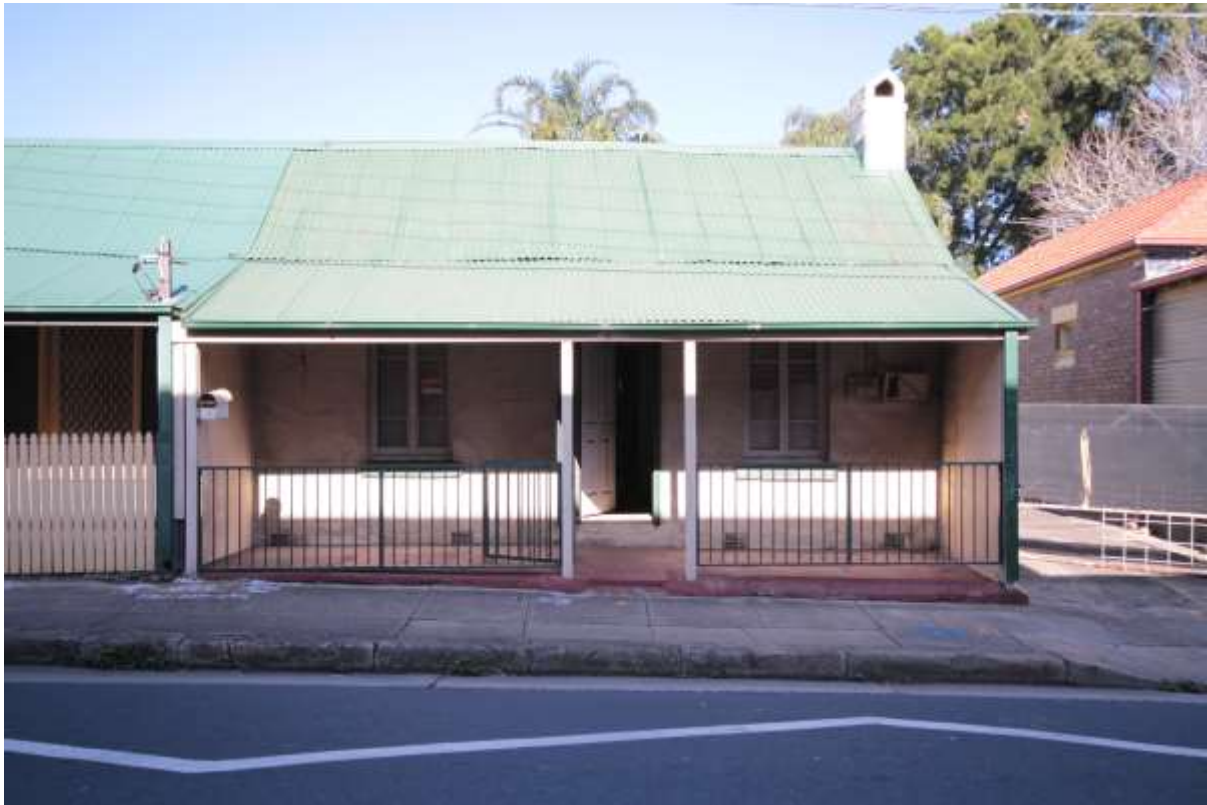
Figure 9. 82 Campbell Street, St Peters.
