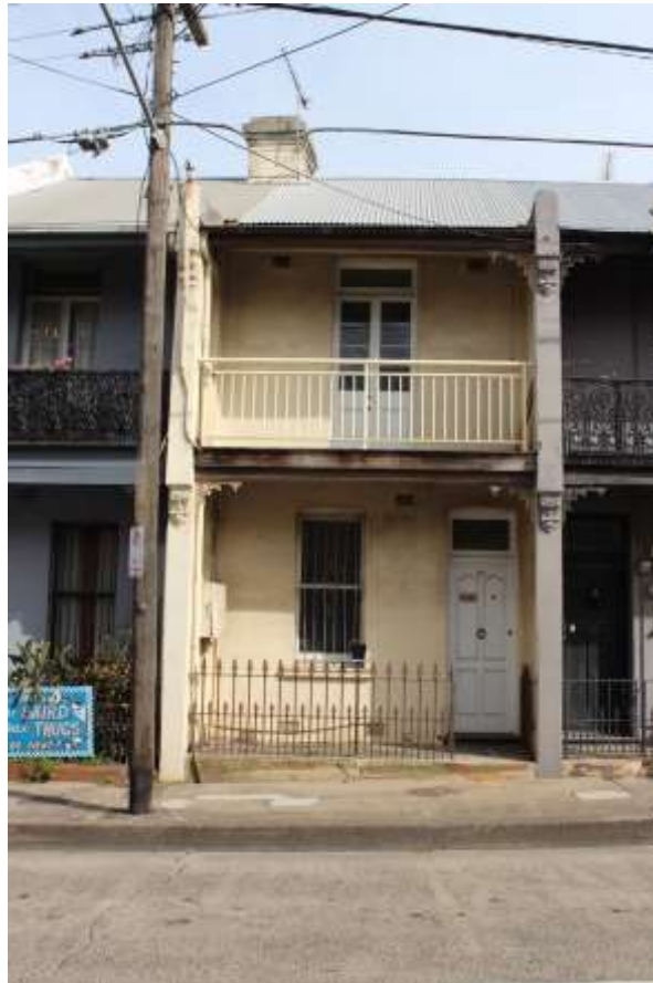
Figure 4. Front façade of 30 Campbell Street, St Peters.
