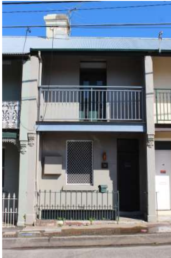
Figure 7. 38 Campbell Street, St Peters.
