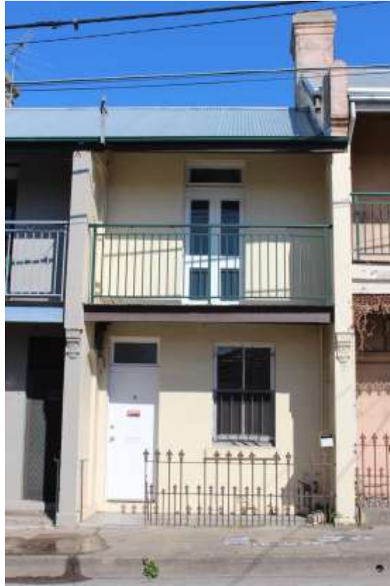
Figure 8. 40 Campbell Street, St Peters.
