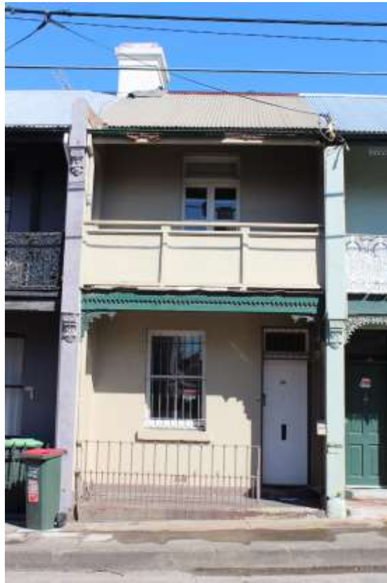
Figure 5. 34 Campbell Street, St Peters.
