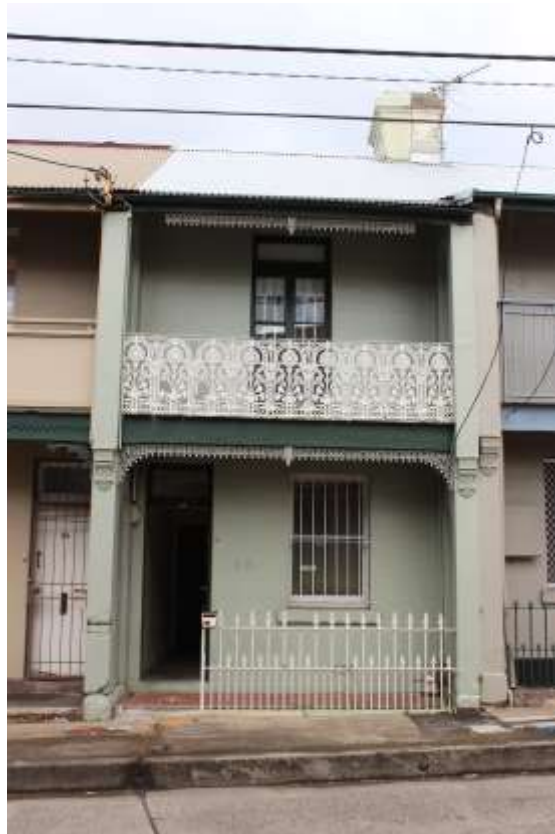
Figure 6. 36 Campbell Street, St Peters.
