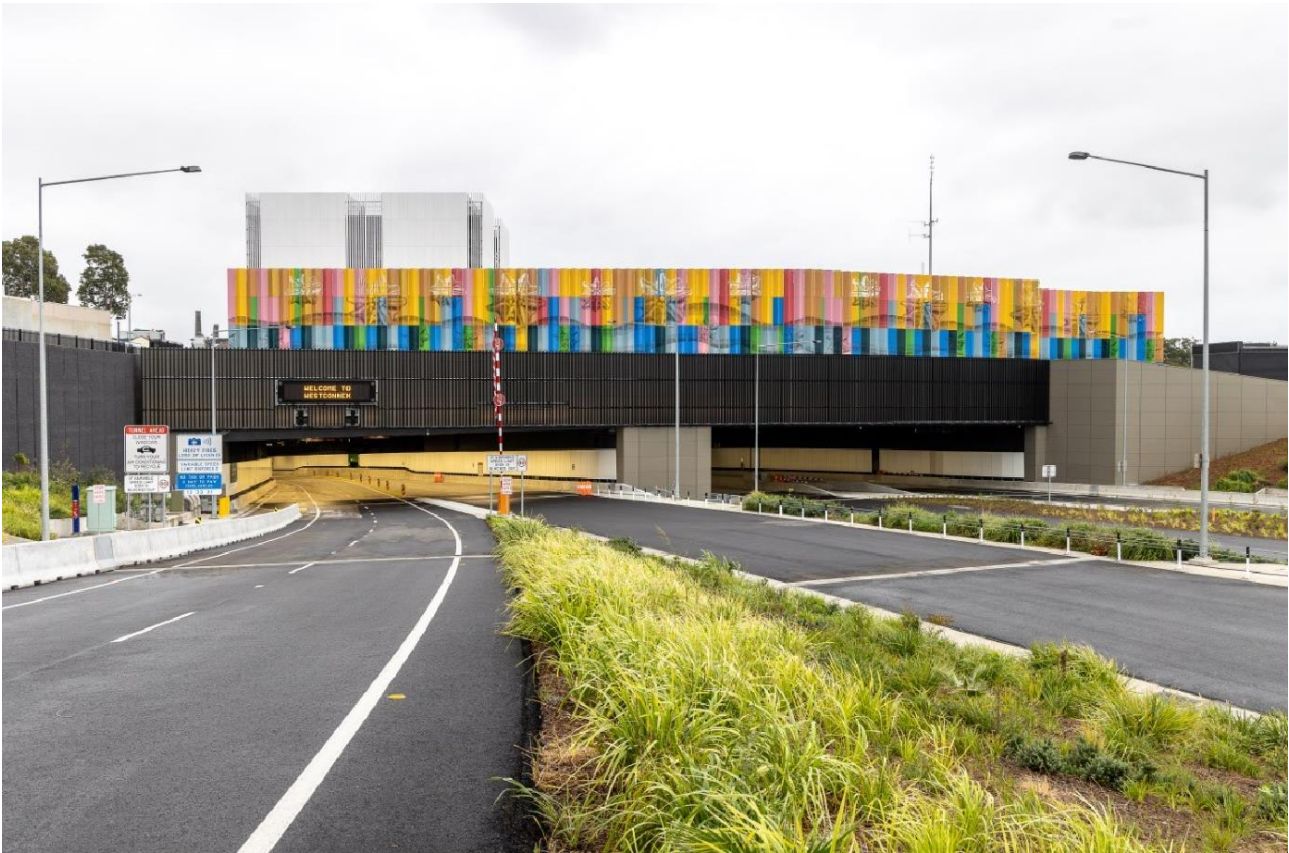
Figure 2-2 Campbell Road Ventilation Facility and tunnel portal
