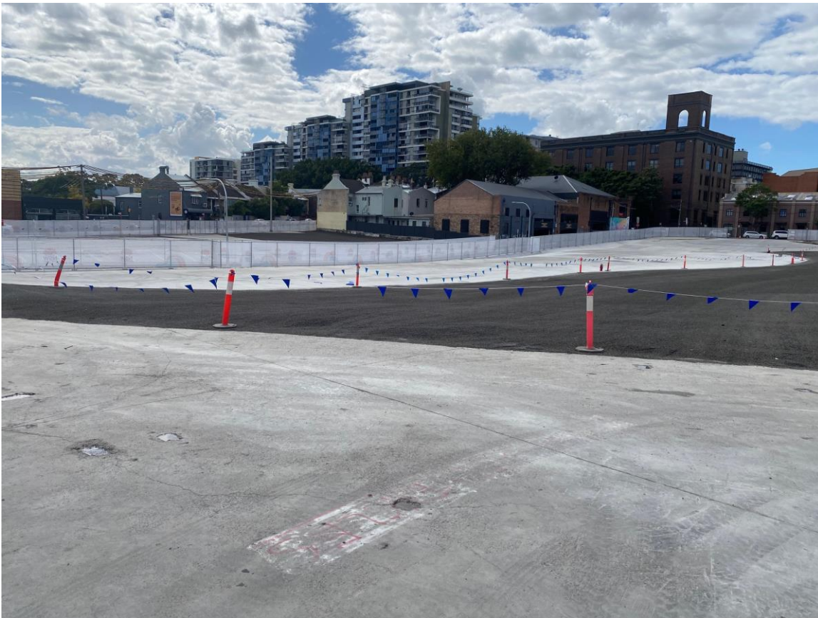
Figure 2-8 Pymont Bridge Road site following reinstatement and demobilisation
