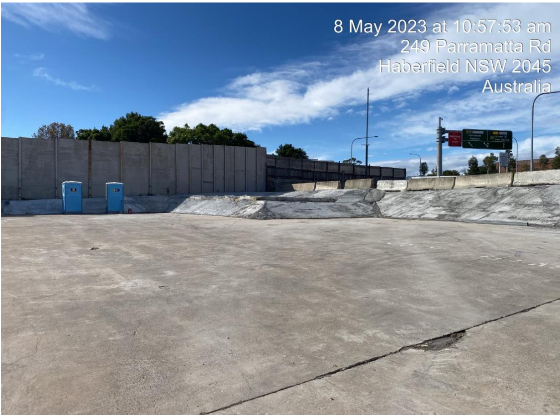
Figure 2-6 Northcote Street site following reinstatement and demobilisation
