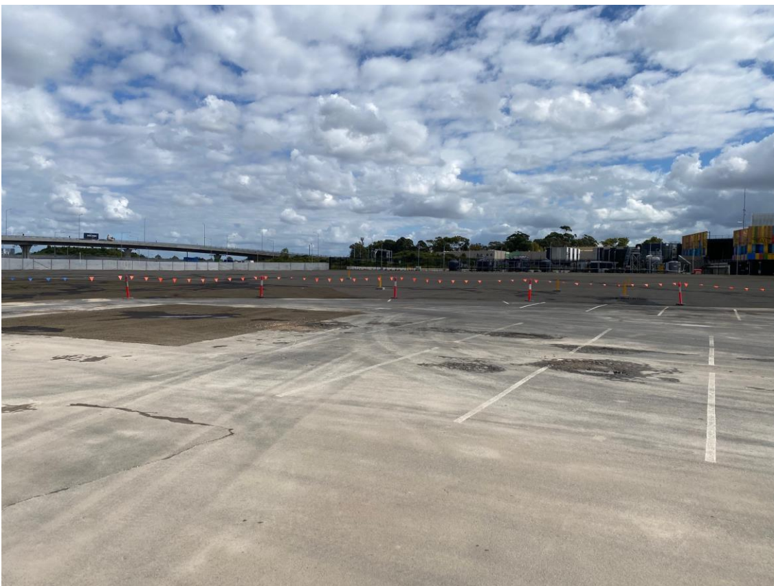
Figure 2-10 St Peters Interchange site following reinstatement and demobilisation
