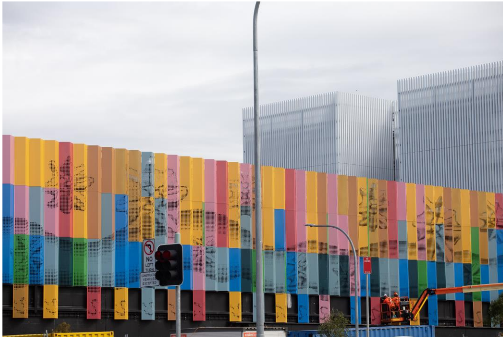
Figure 2-4 Ventilation and substation cladding, St Peters, April 2022
