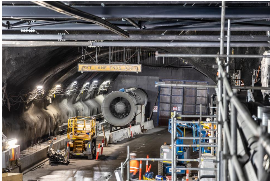
Figure 2-1 – M&E works underway at Haberfield, May 2022.
