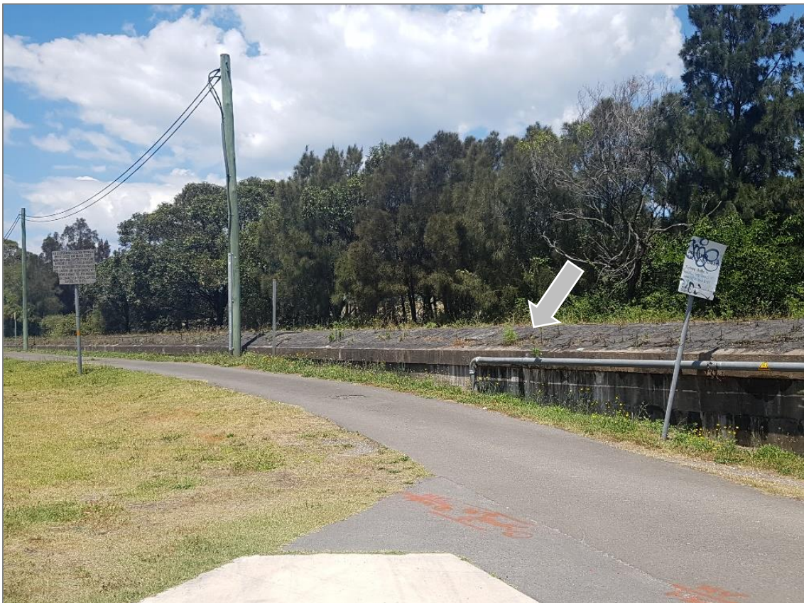
Plate 1 – Arrow notes SWSOOS, note the ground level change.
