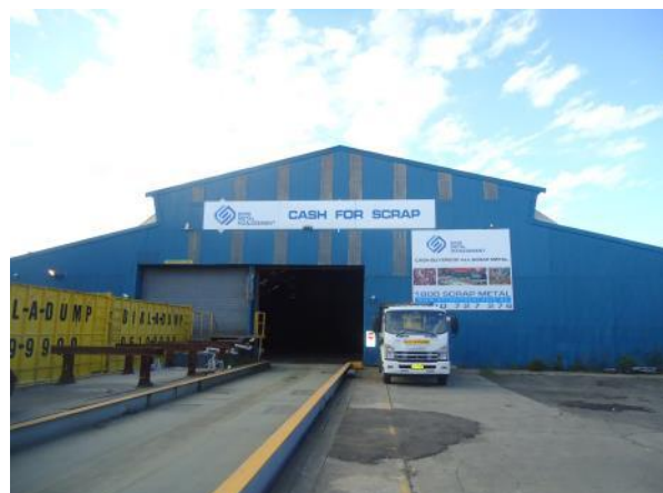
Plate 84 Rudders Bond Store from Burrows Road entrance. View north.
