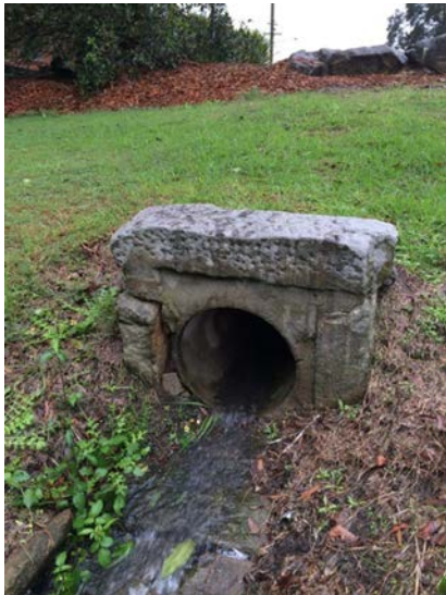
Plate 8 Sandstone and concrete drain
