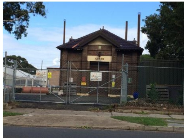
Plate 55 Huntley Street Sewage Pumping Station.
