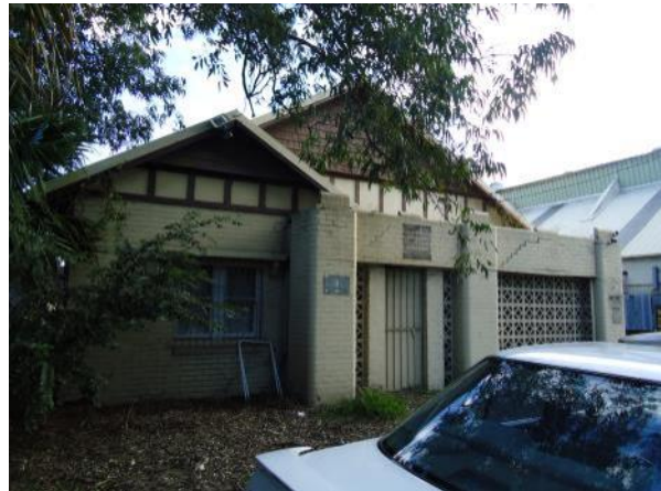
Plate 88 Building associated with the Rudders Bond Store. View south west
