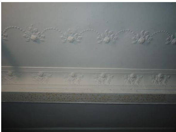
Plate 89 Building associated with the Rudders Bond Store. Interior showing moulded plaster ceilings in hallway.
