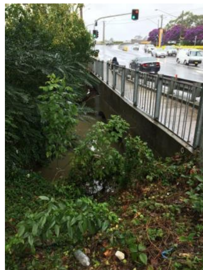
Plate 12 Downstream side of culvert from northern bank
