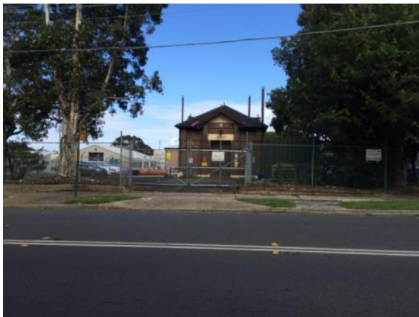
Plate 54 Huntley Street Sewage Pumping Station.
