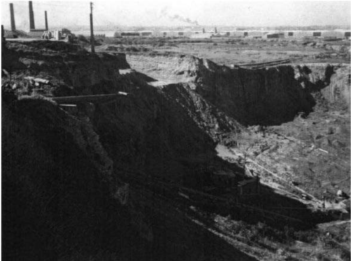
Figure 17. Looking down into the Austral pit which was shared by The Central Brick and Tile Co Pty Ltd whose four chimney stacks and kilns can be seen to the left. Note: Barwon Park House can be seen in front of the four chimney stacks. Date unknown, but is pre-1953. (Source: Ron Ringer (2008) “The Brickmasters 1788-2008”, Dry Press Publishing, p. 251)
