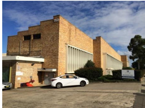
Plate 78 Former Westpac Stores. View south.
