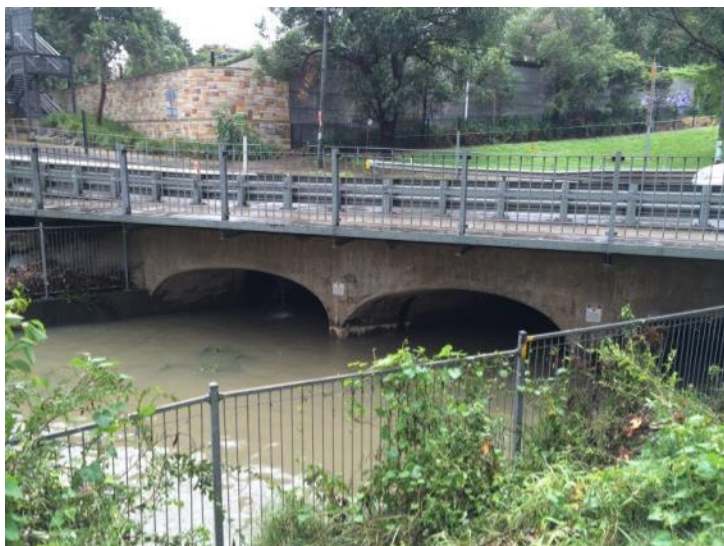
Plate 11 Culvert and footway from southern bank
