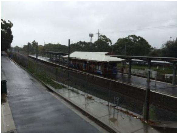
Plate 4 Overview of Bexley North Railway Station. View north west
