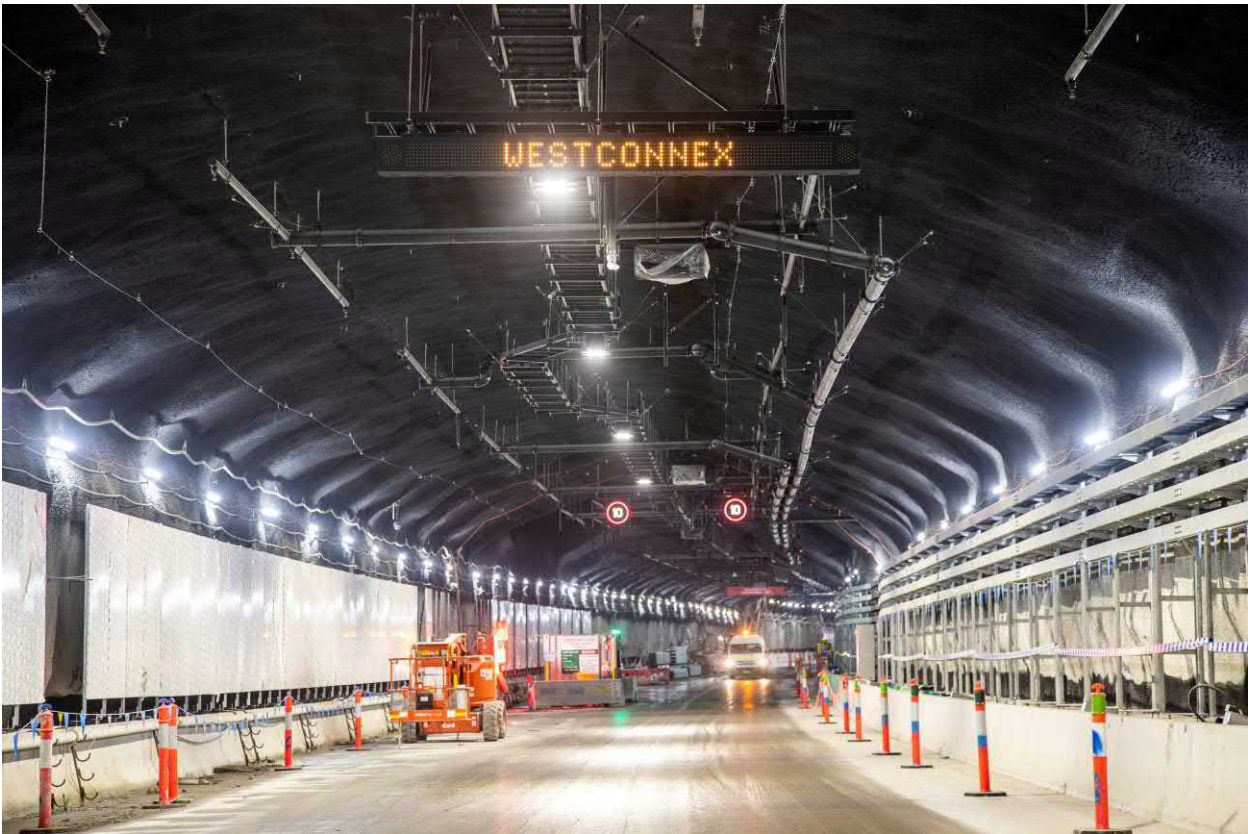
Figure 2-2 – Ongoing M&E works at SPI in October 2021
